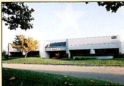
Pictured is dB Control's new 16,000 sq. ft. facility (Photo courtesy of dB Control)
